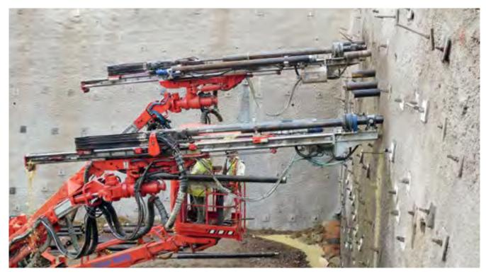
1. For drilling, the starter unit with drill bit is assembled onto the drill boom together with the first extension tube, the adapter, and the drill rod.
