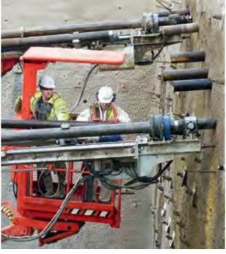
The next drill rod with extension tube is connected to the previously installed pipe and the drilling process is continued. Reloading AT – Automation Unit (extension tube and drill rod).
